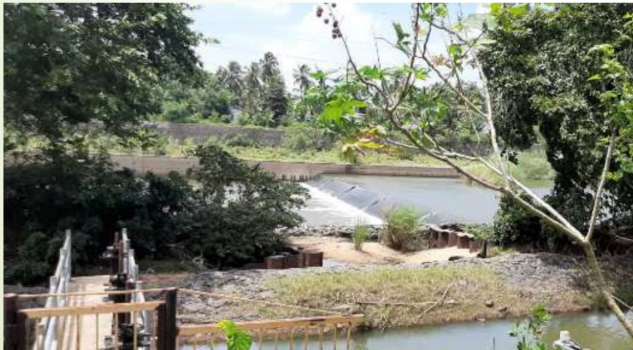
Completed the salinity barrier in 2017
