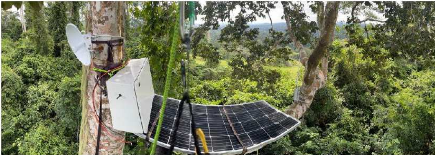
Solar panel to support sensor network established in Bouamir by FieldKit team.
